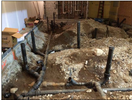
Underground Sanitary & Grease Waste Piping Roughed In and Tested
