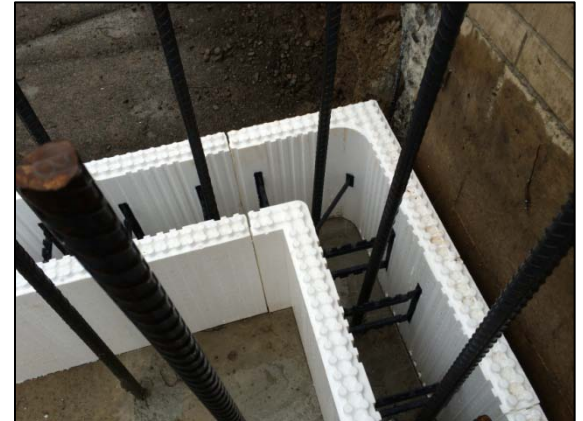
Installing Insulated Concrete Forms (ICF)
