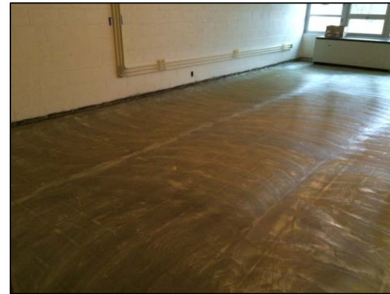
Subfloor Surface Prep and Adhesive
