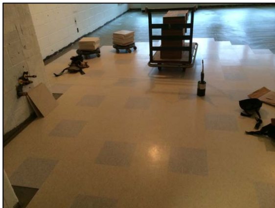
Installing tiles
