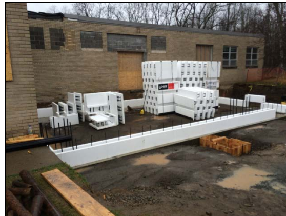
Installing Insulated Concrete Forms (ICF)
