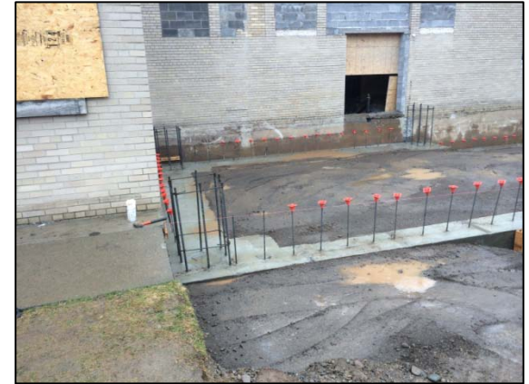
Footers Stripped and Backfilled
