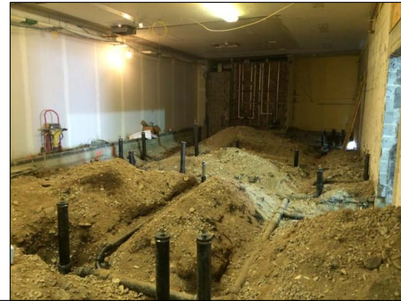
Underground Sanitary & Grease Waste Piping Roughed In and Tested
